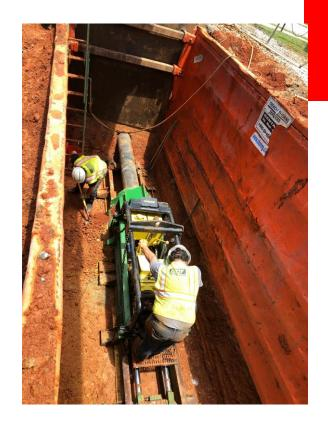
Jack and Bore to 10<sup>th</sup> Street Manhole for Sanitary Sewer at New Addition
